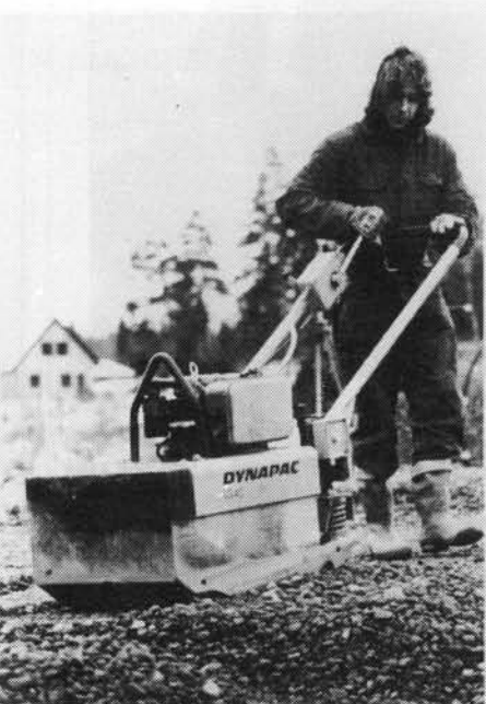
DYNAPAC LG 40 vibrating plate is compacting a gravel base course. It weighs 380 Kg fitted with a Hatz diesel engine. Other engine options are available.
